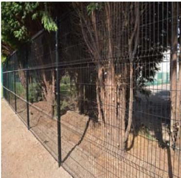
Trifen Engineering is a UK stockist for Paramesh 3M system. The panel construction features galvanised horizontal and vertical rods of 5mm diameter. These are resistance welded at the intersection points to form a 200mm x 50mm mesh pattern.
